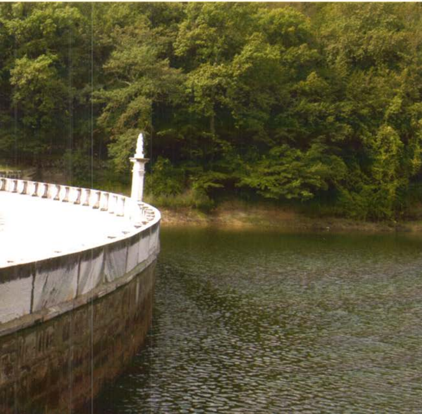
Sultan Mahmud II Dam
