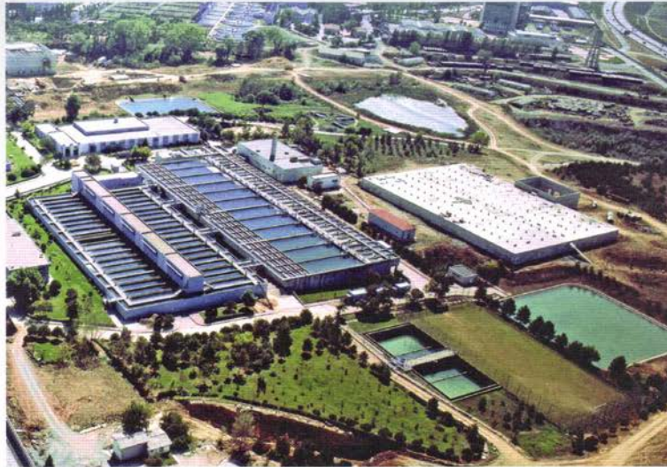
Kağıthane Water treatment facility
